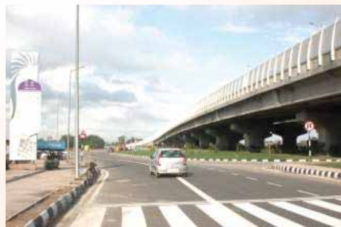
DDA Flyover on NH-24 near Commonwealth Games Village
